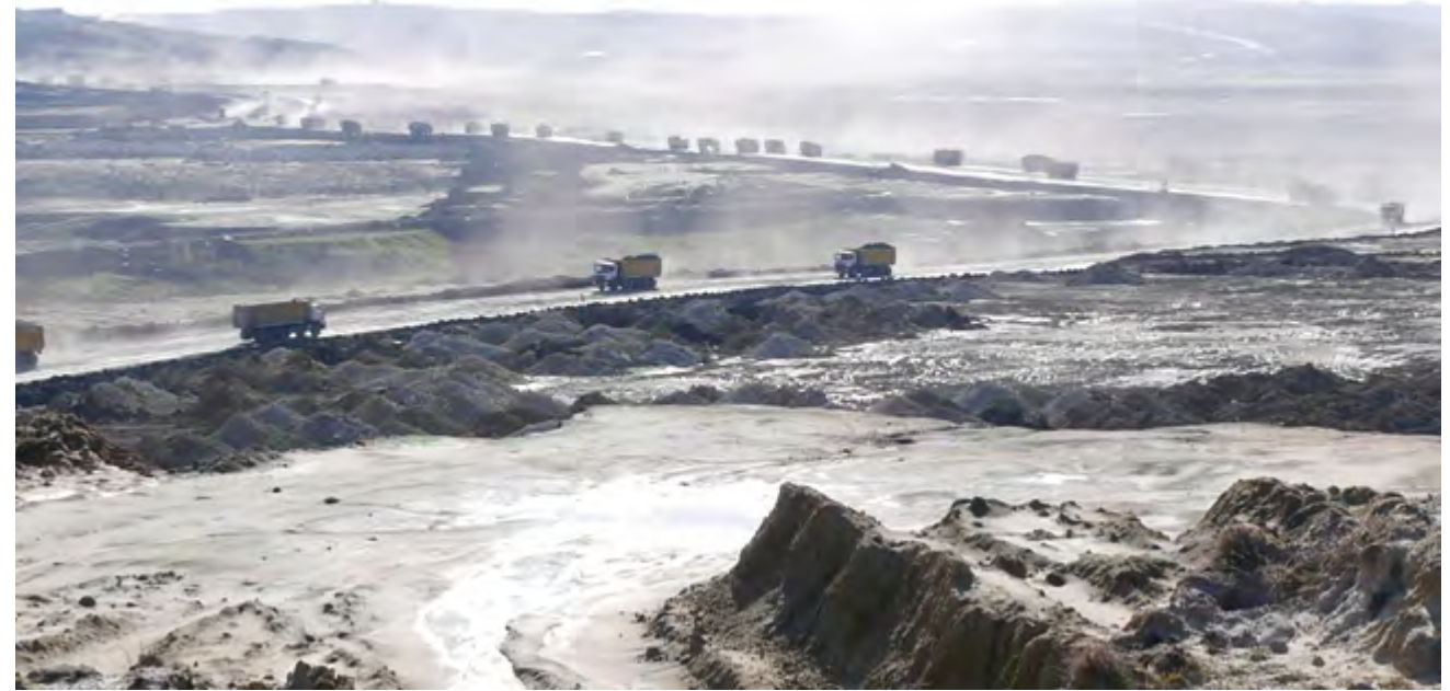
Construction site, Istanbul 3rd airport (Source: Still frame, Northern Forests, TR/D 2020, HD, 86min, Julia Lazarus)
